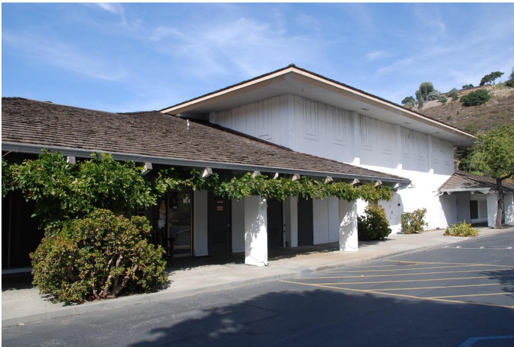
Figure 10. 2019 view rear of former cinema and shopping center, view northwest. Source: Page & Turnbull
